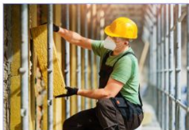
Renovation of public buildings
