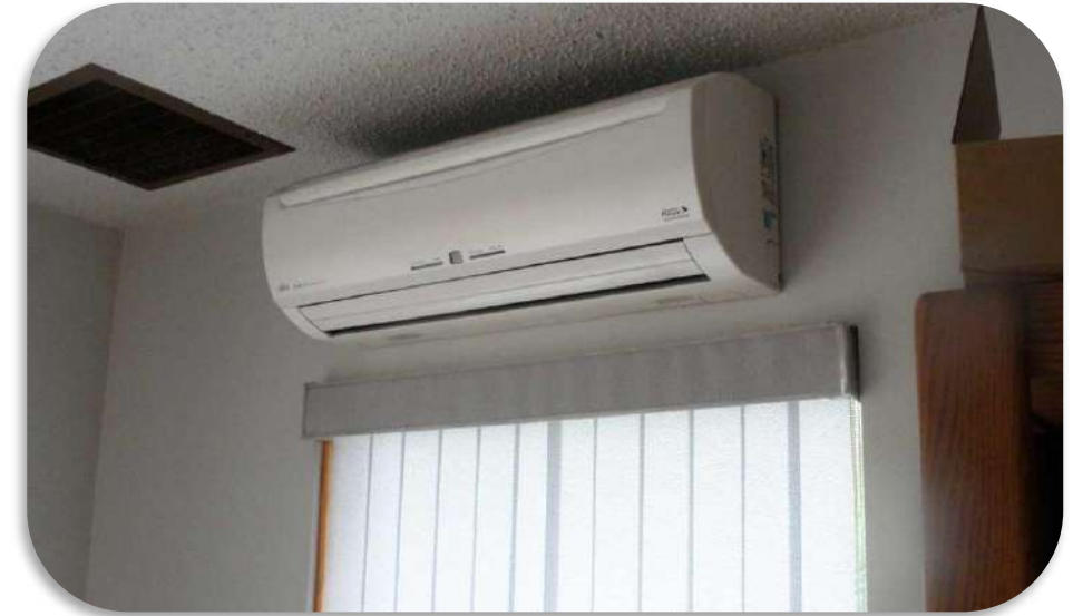
The indoor unit of an Air-source heat pump
